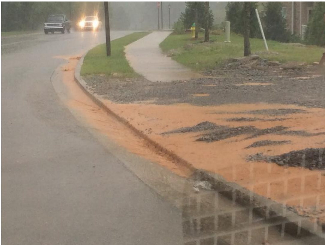
Water and mud runoff onto Wellsley Park Rd., Aug. 18, 2014
