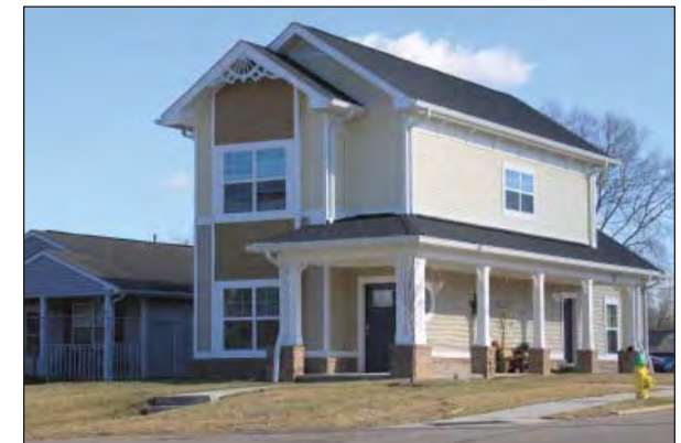
Infill housing has made a positive impact in the sector.
