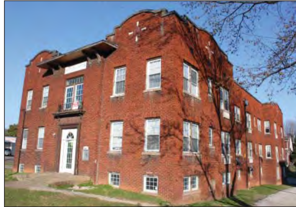
Aston Apartment building
