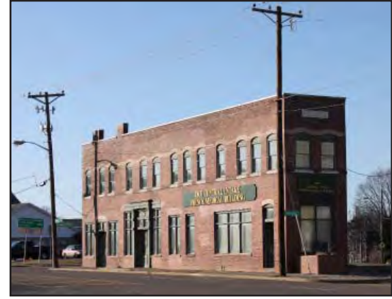
1601 Western Avenue - Prince Building (c.1900)
