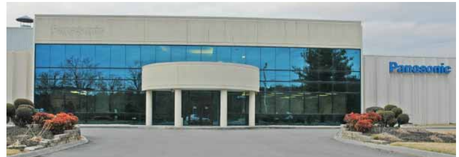
Almost all of the manufacturing and distribution facilities are in the Fork of the River area.
