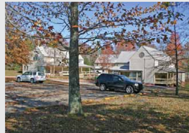
Office, retail and other facilities (Big South Folk) that are an example of designing with traditional materials and at an appropriate scale for larger rural commercial development
