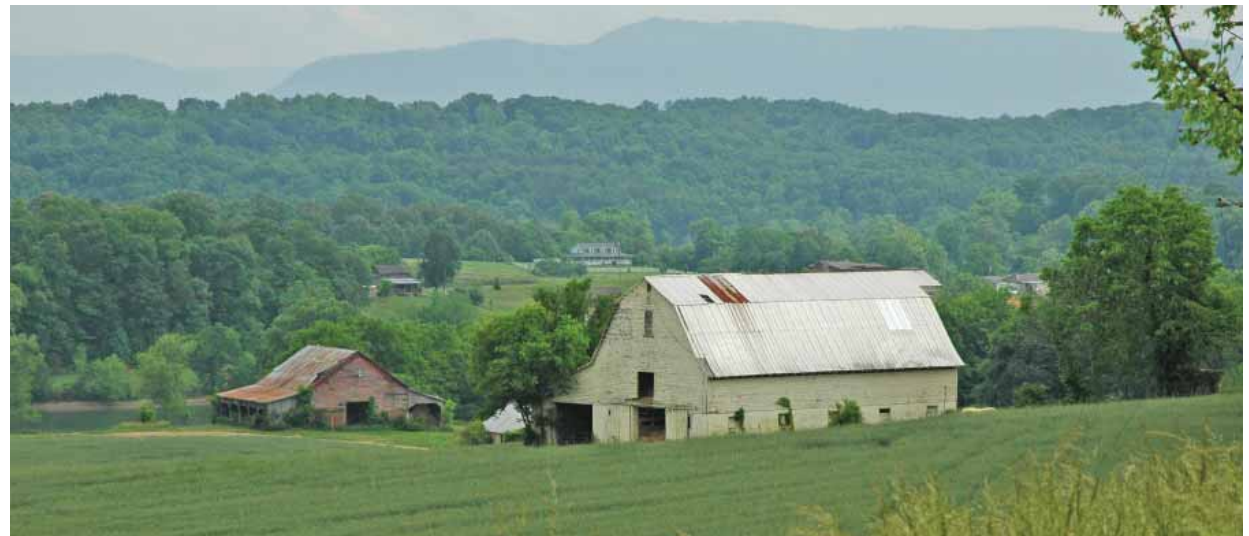
The designated Rural Area is 55 percent of the sector’s land area.
